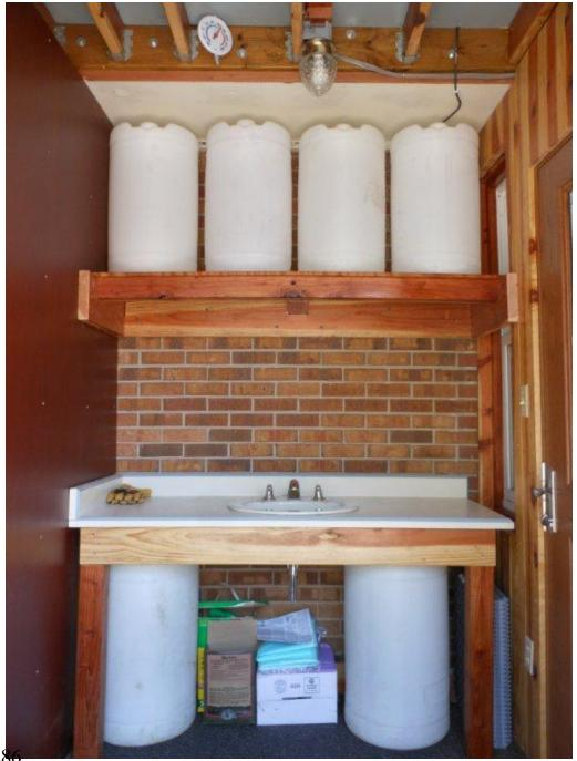
•<u>Airlock</u> to Greenhouse – •Dual Purpose: Doubles as <u>Potting</u> <u>Shed</u> – with water based <u>thermal</u> <u>storage</u>.
