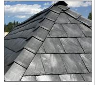
RoofsByJohnson.com. The cost is more than twice that of a conventional roof, but it comes with a 50year warranty against damage from up to 2" hail with no pro-rating and no deductible. The company installed a Euroshield roof in Golden's Amberwick subdivision after a 2017 hail storm. Those roofs survived two subsequent hail storms without any visible damage.
