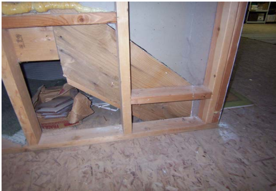
Standard framing on structural wood floor over crawl space.
