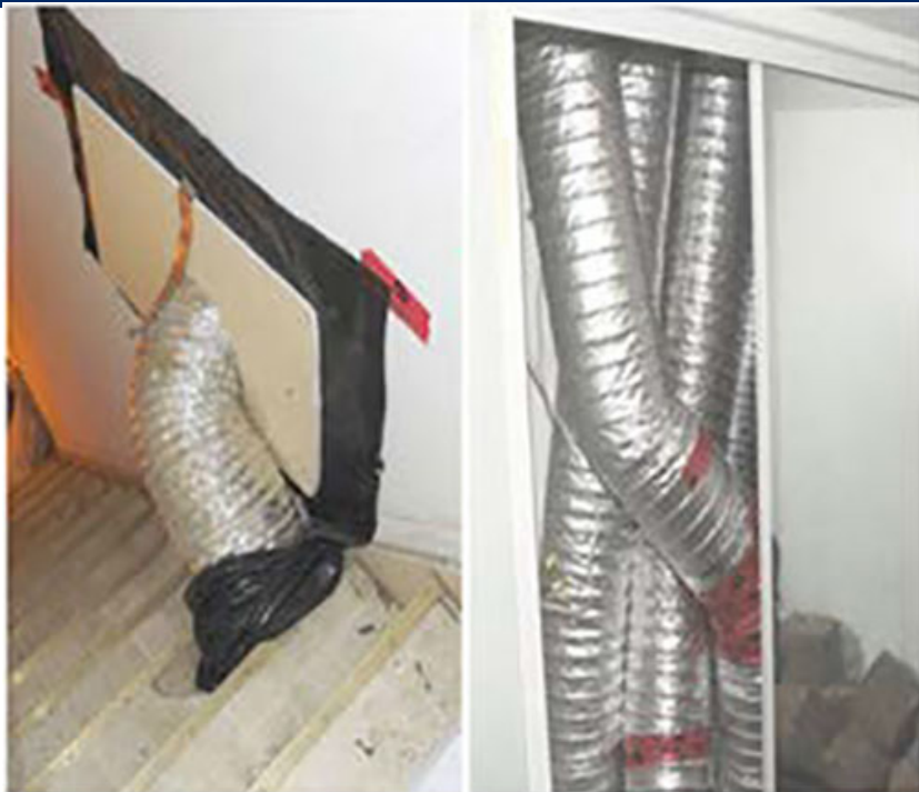
FIGURE 2. DO-IT-YOURSELF VENTILATION IN A COLORADO GROW HOUSE
