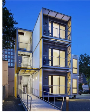
IndieDwell, a Boise-based company, offers this 2-bed unit built from an 8'x40' shipping container for $50,000. Setup time is 18 days.
